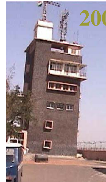
Kandla port building after 2001 Bhuj earthquake
