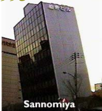
Building in Kobe after 1995 earthquake
