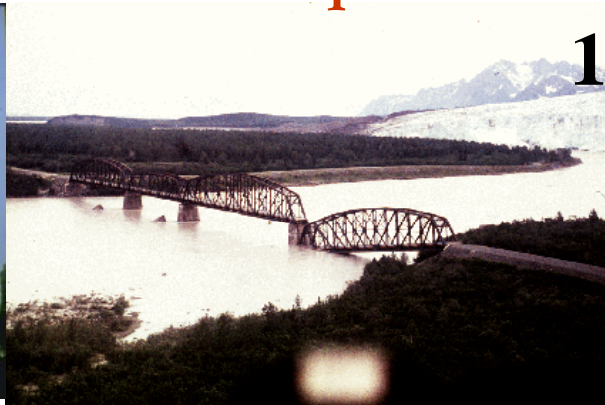
Million Dollar Bridge after 1964 Alaska earthquake
